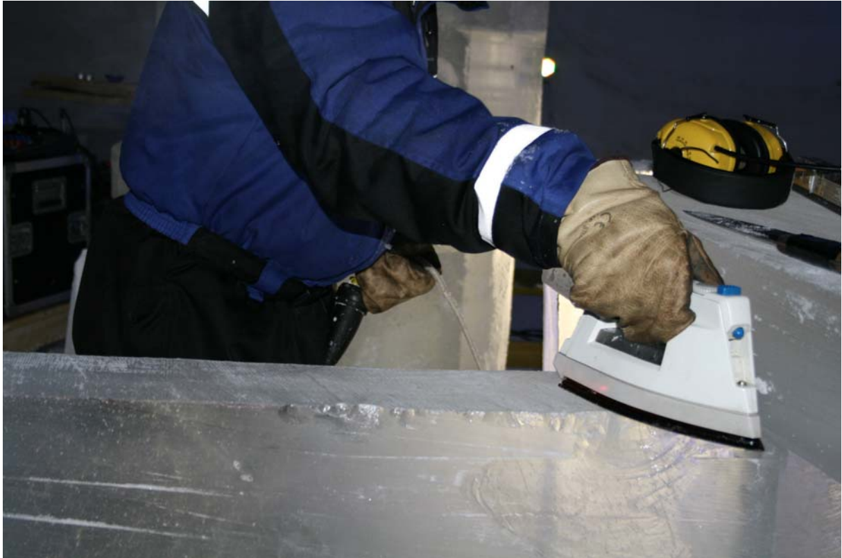
A local craftsman demonstrates use of an iron to make the ice smooth and crystal clear, Lainio 2007
