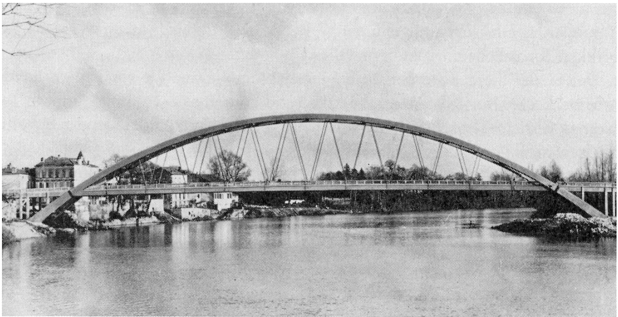
Fig. 61e. The Castelmoron Bridge built in France in 1933
