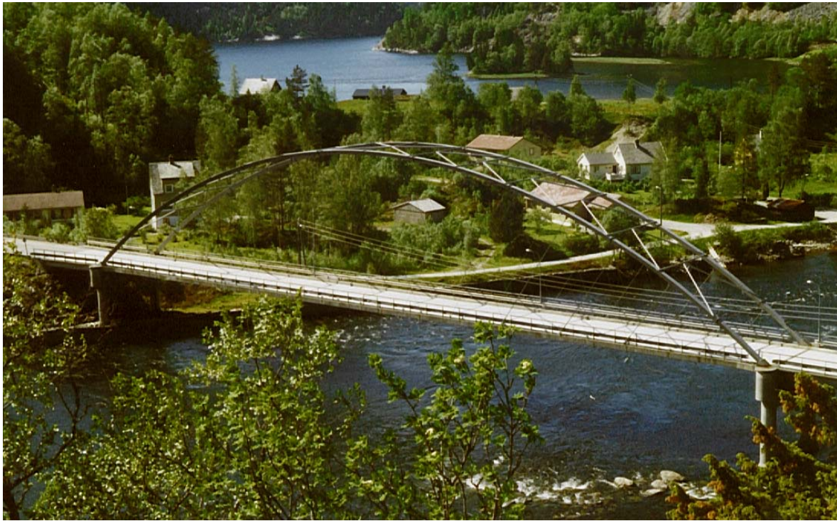
Fig. 7. Bolstadstraumen Bridge. The main span is 84 metres.
