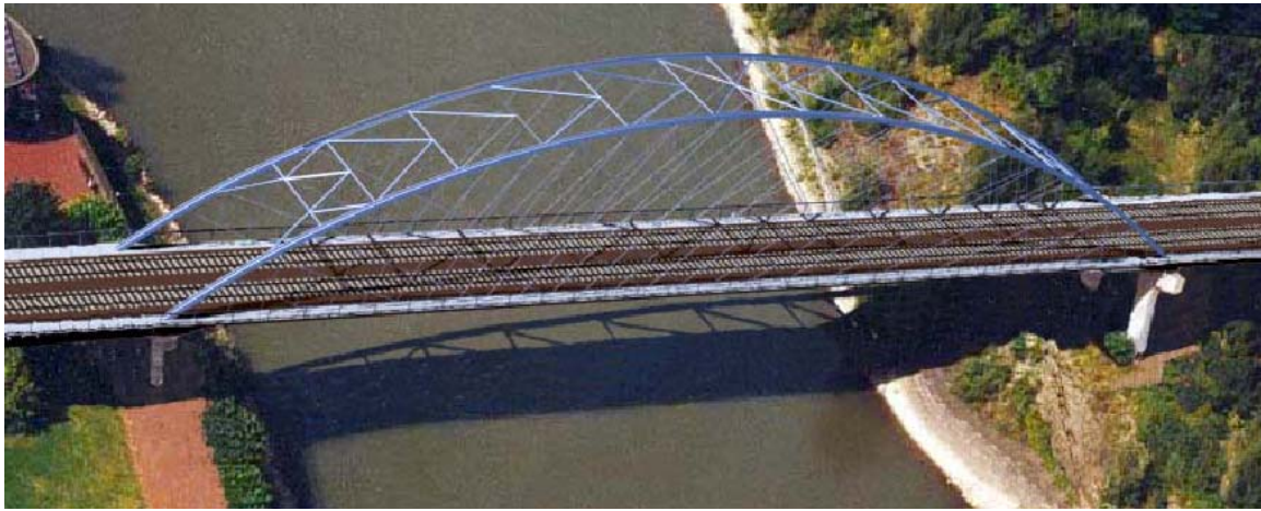
Fig. 40e shows a two track railway bridge spanning 100 m designed by Brunn and Shanack
