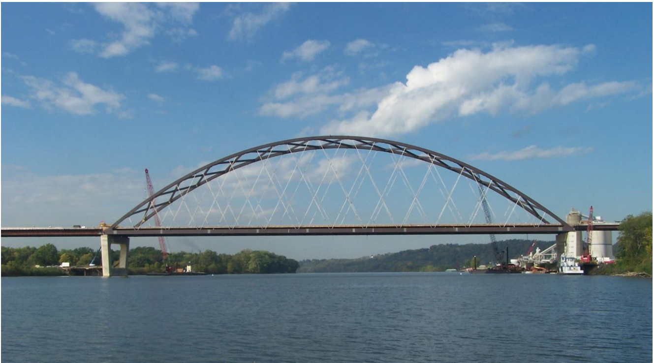
Fig. 54. Blennerhassett Bridge over the Ohio River in the USA. Span 268 m
