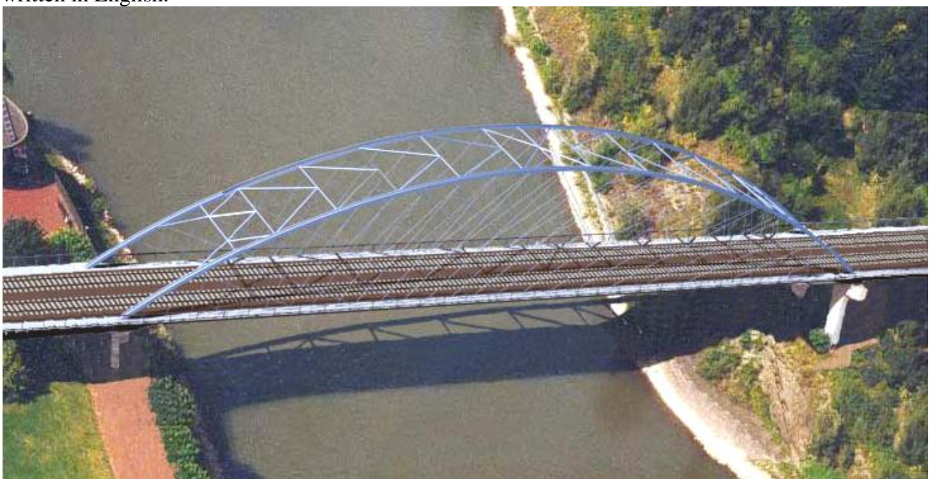
Fig. 36. A double track railway bridge designed in 2003 by Brunn and Schanack.
