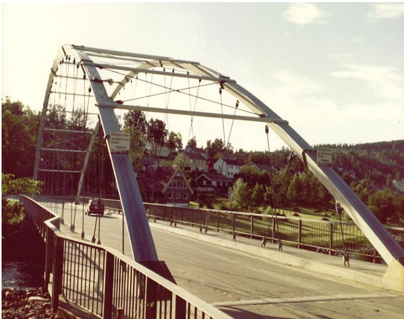
Fig. 5. Network arch at Steinkjer. Span 80 m.
