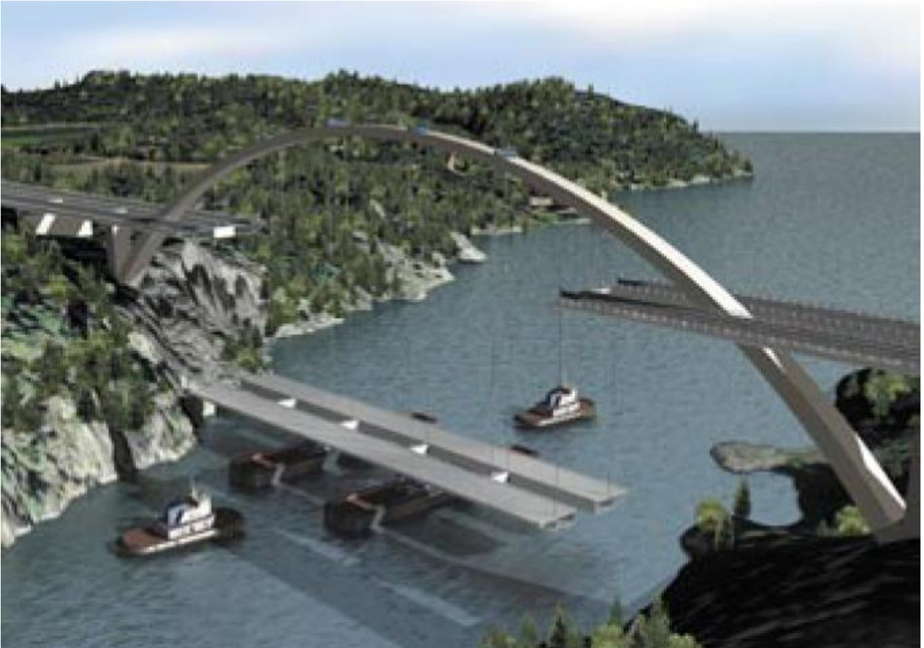
Fig. 58 Closing the Svinesund Bridge.
