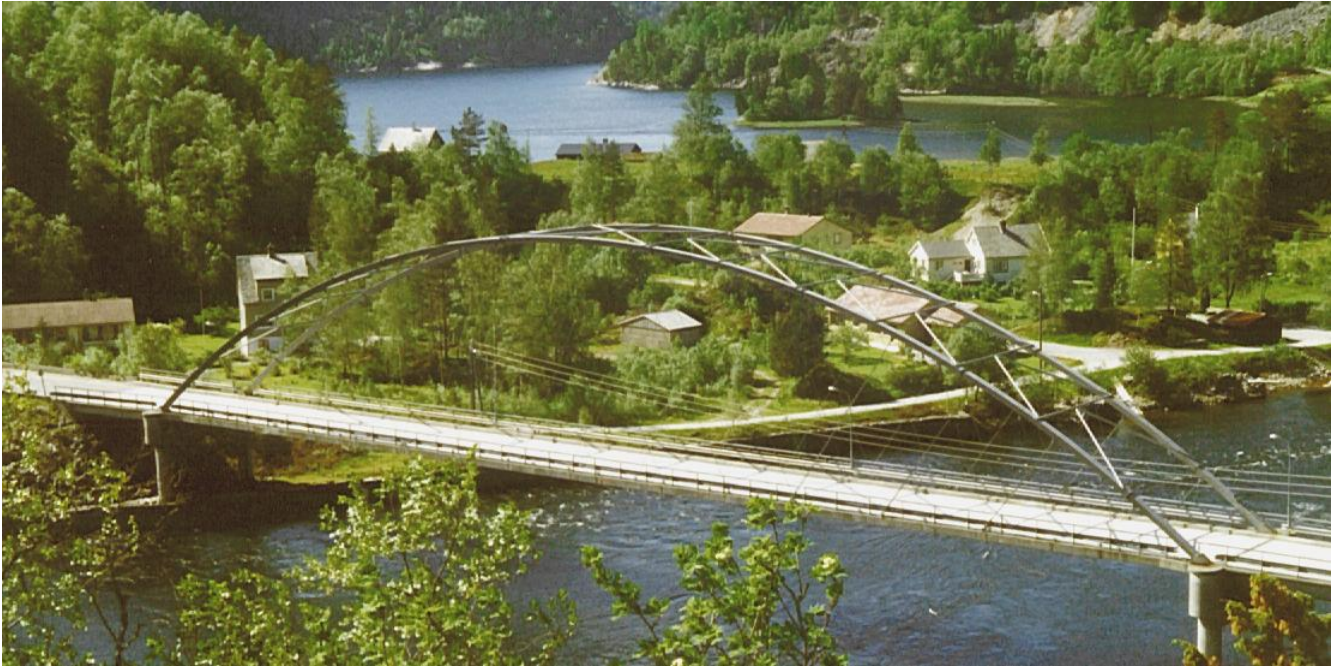
Fig. 1. Bolstadstraumen Bridge has a span of 84m.
