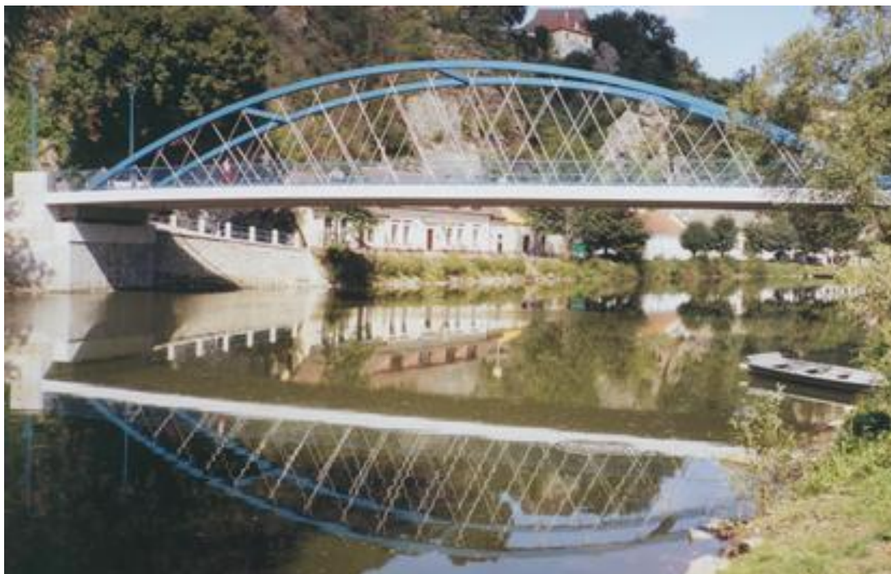
Fig. 46. The Bechyne Bridge built in 2004. Span 41 m.
