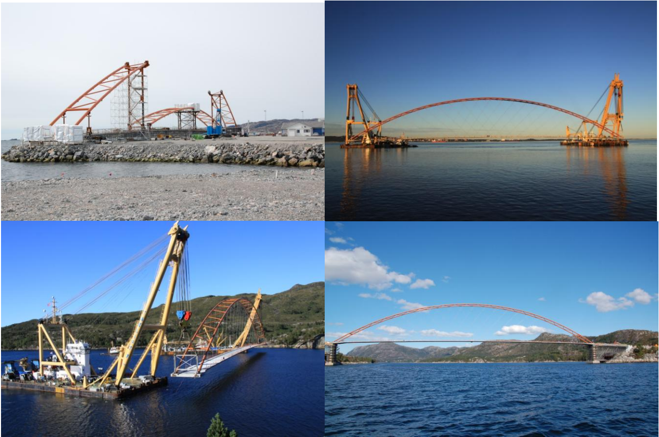
Fig. 61. Four stages in the erection of the Brandanger Bridge.
