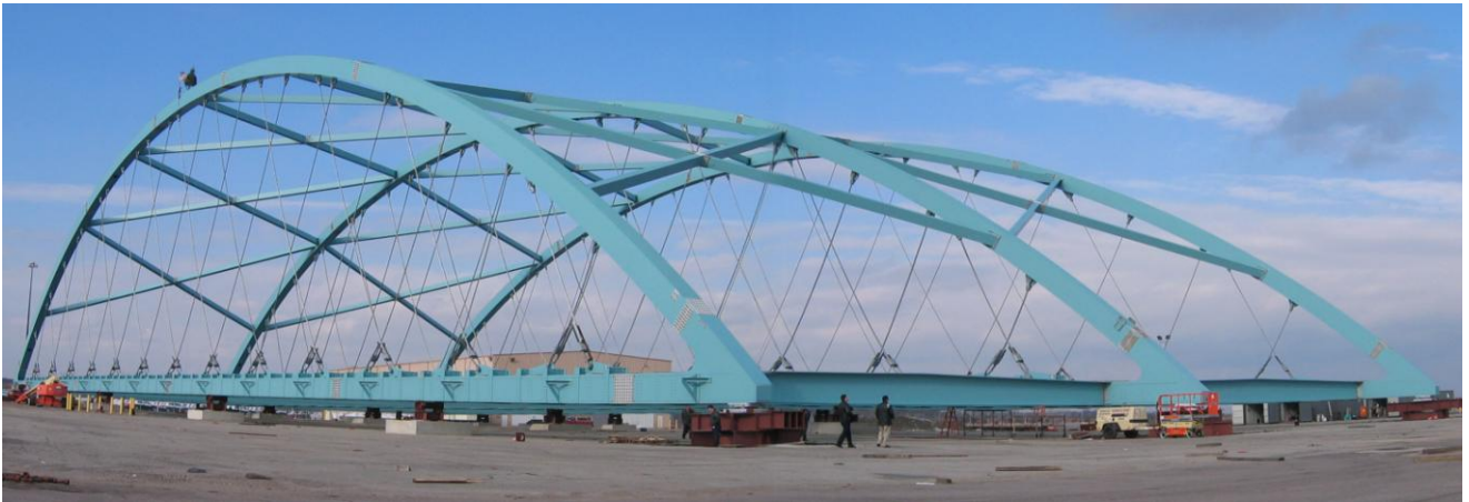
Fig. 50. The steel skeleton of the network arch in Providence ready to be moved.
