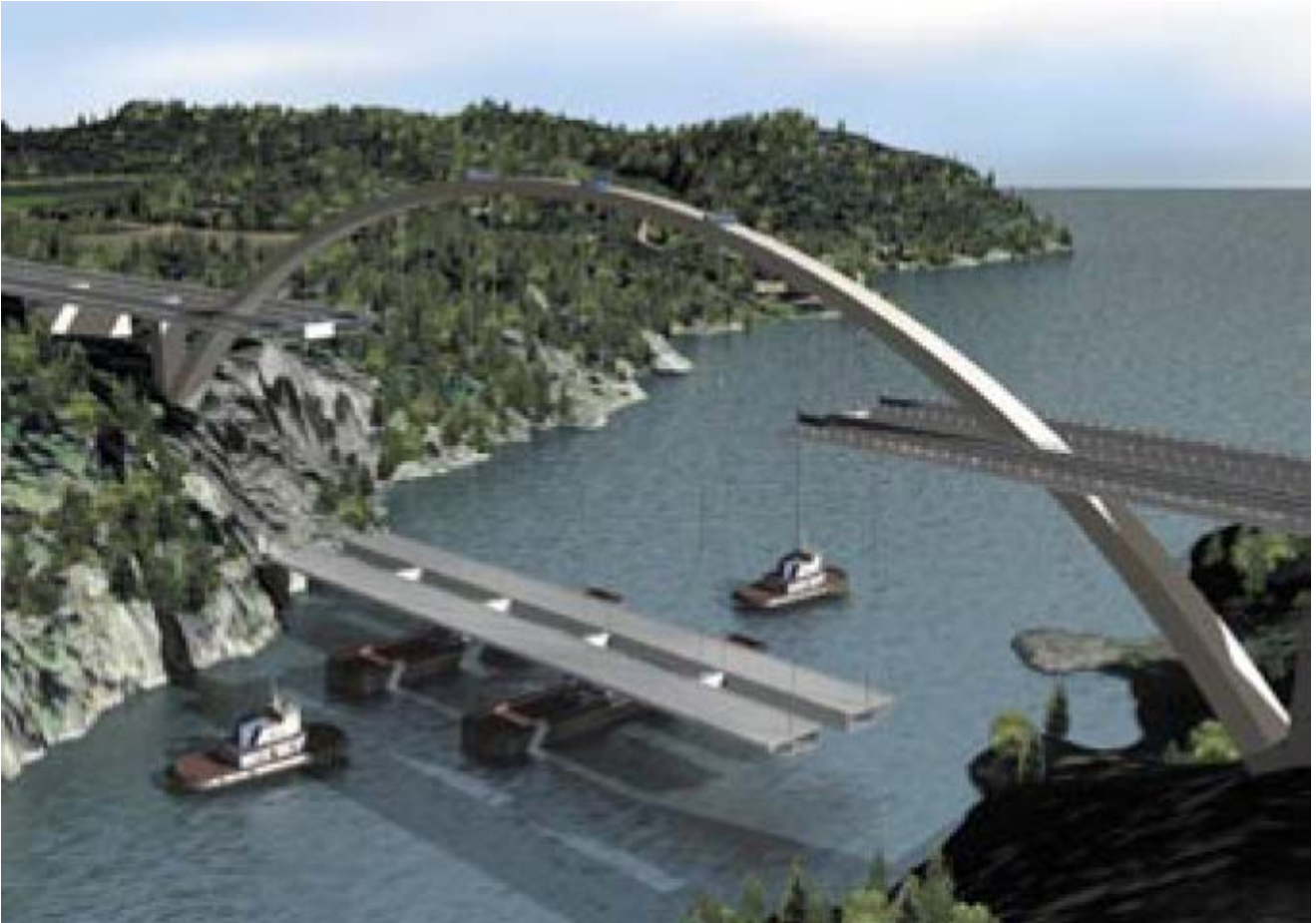
Fig. 58 Closing the Svinesund Bridge.
