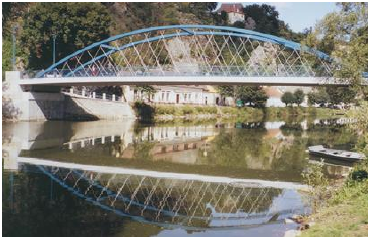
Fig. 46. The Bechyne Bridge built in 2004. Span 41 m.
