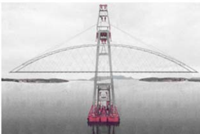
Fig. 33. Lifting the steel skeleton of a network arch with a floating crane.
