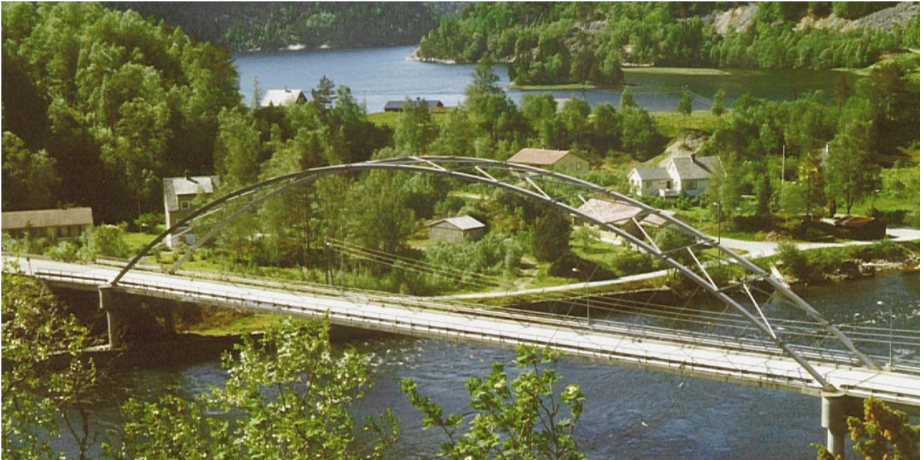
Fig. 1. Bolstadstraumen Bridge has a span of 84m.
