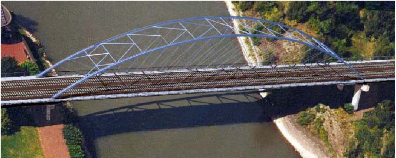
Fig 50. Two-track railway bridge spanning 100 m. [Brunn and Shanack 2003].
