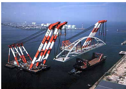
Fig. 39. Lifting of the Shinhamadera Bridge.
