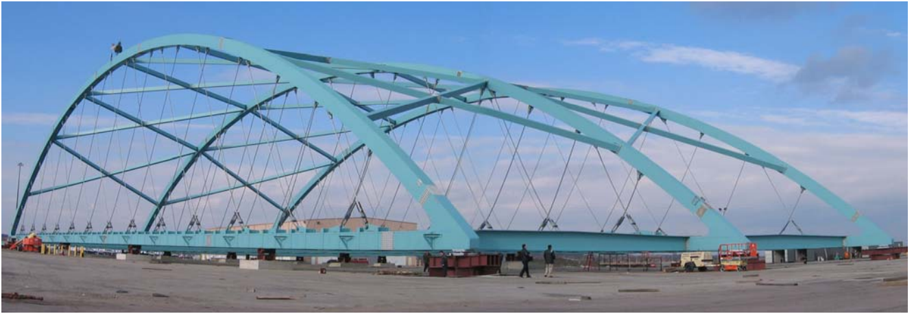
Fig. 69. The steel skeleton of the network arch in fig. 68 before it is floated to the site.
