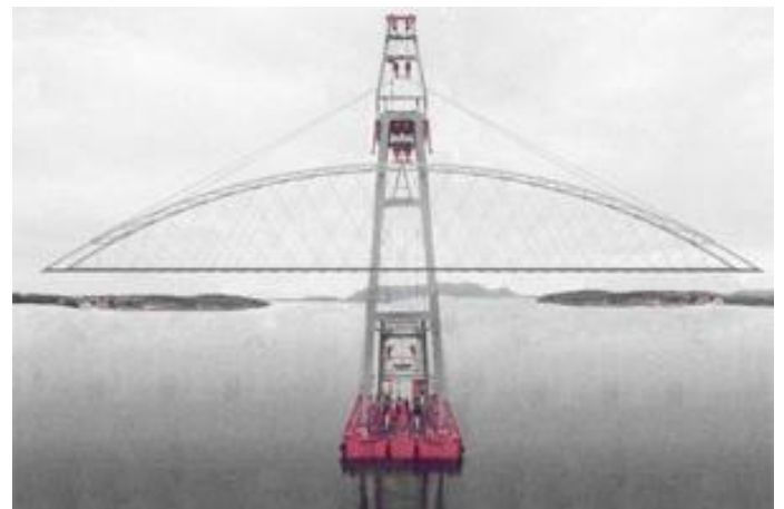
Fig. 13. Lifting the steel skeleton of the bridge in fig. 4
