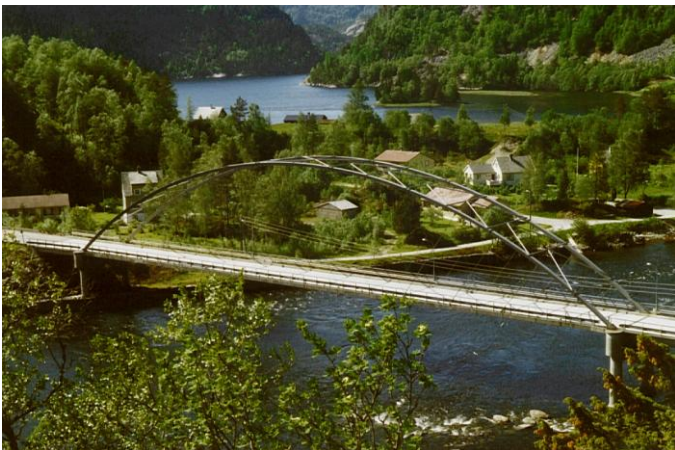
Fig. 1. Bolstadstraumen Bridge in western Norway.
