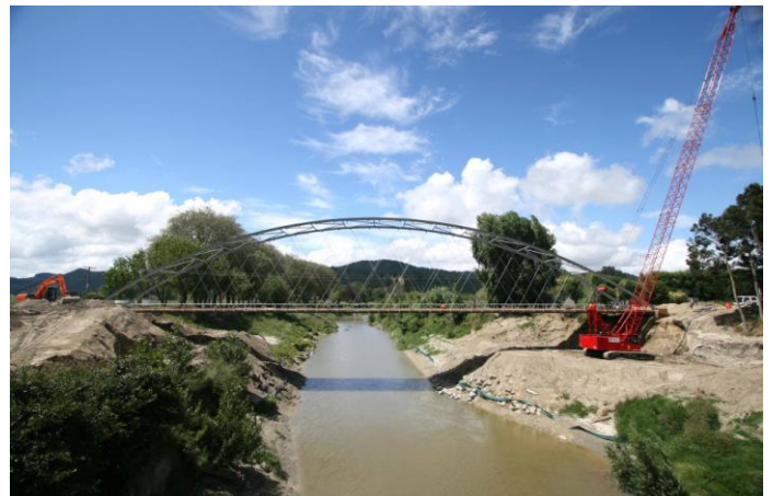
Fig. 2. Mangamahu Bridge, New Zealand.
