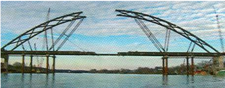
Fig. 19. Erection of Blennerhassett Bridge. The last beams in the tie is about to be put in.
