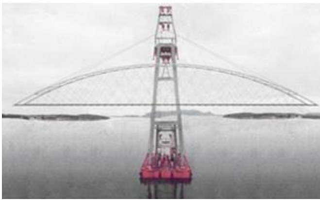
Fig. 35 shows lifting of a steel skeleton
