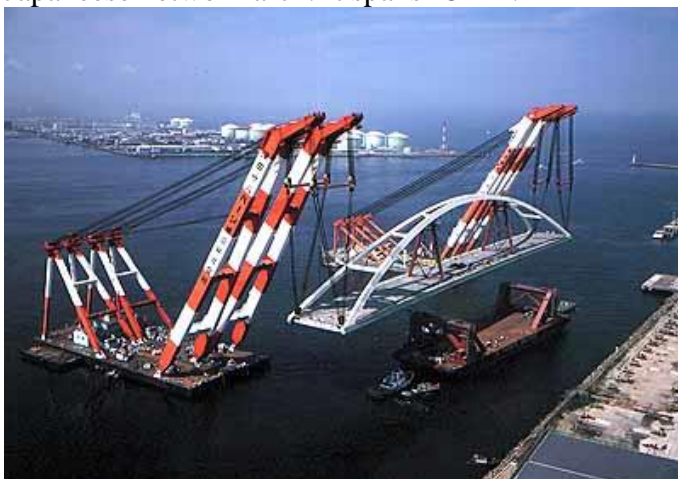
Fig. 29. Lifting of the Shinhamadera Bridge. The tide helped in putting the main span in place.
