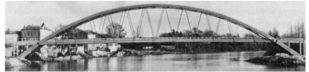
The longest Nielsen bridge. Castelmoron 1933. Span 145 m.
