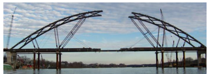
Fig. 58. Arch erection
