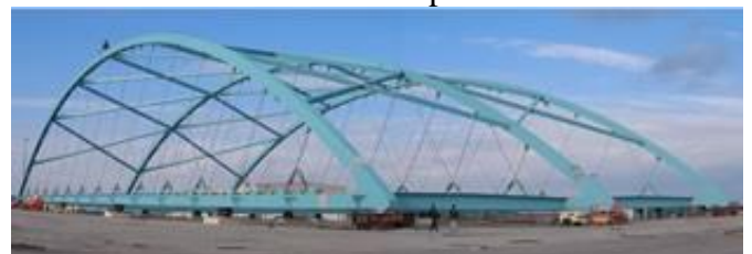
Fig. 52. Steel skeleton for the bridge in Rhode Island
