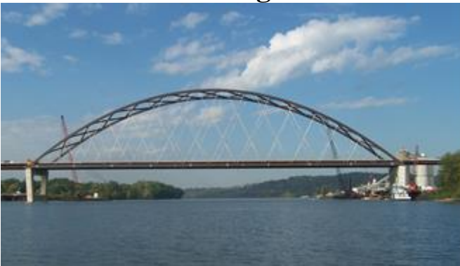
Fig. 55. The world's longest network arch. Span 268m
