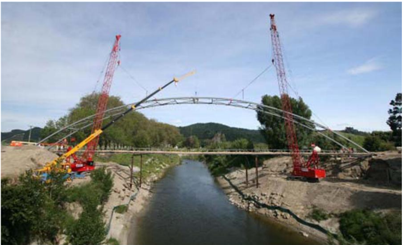
Fig. E8. Method for lifting the steel skeleton of the Mangamahu Bridge in place. Span 86 m.
