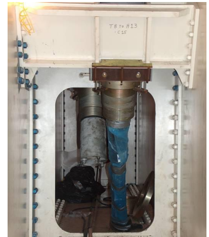
Fig. 6 – Cable Anchorage in Tie Girder
