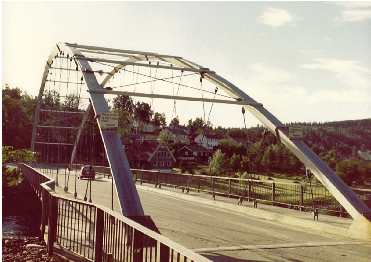
Fig. 2. Bridge at Steinkjer, Norway, opened in June 1963.
