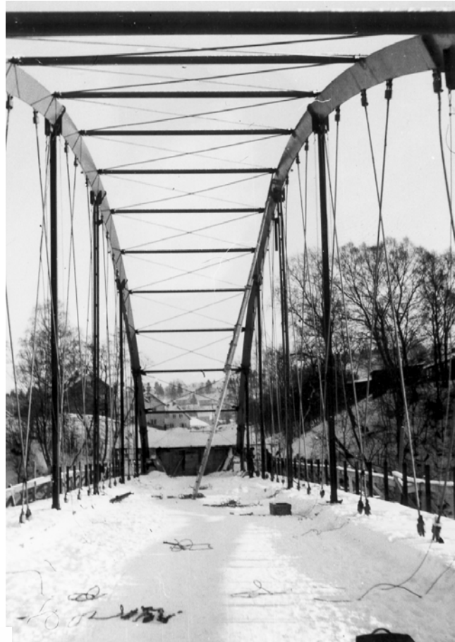
Fig. 4. Erection of the arch of the Steinkjer Bridge.
