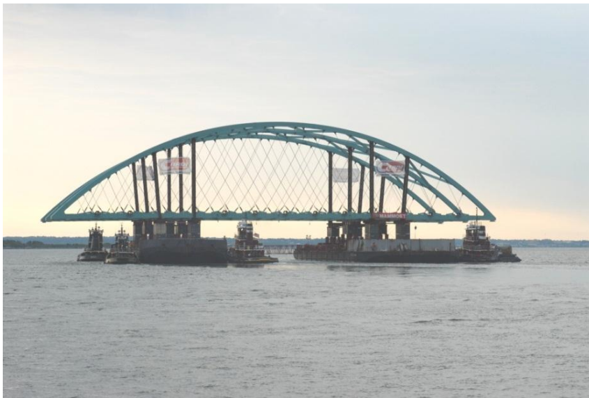
Fig. 30. The main span in the Providence network arch was assembled 19 km from the site
