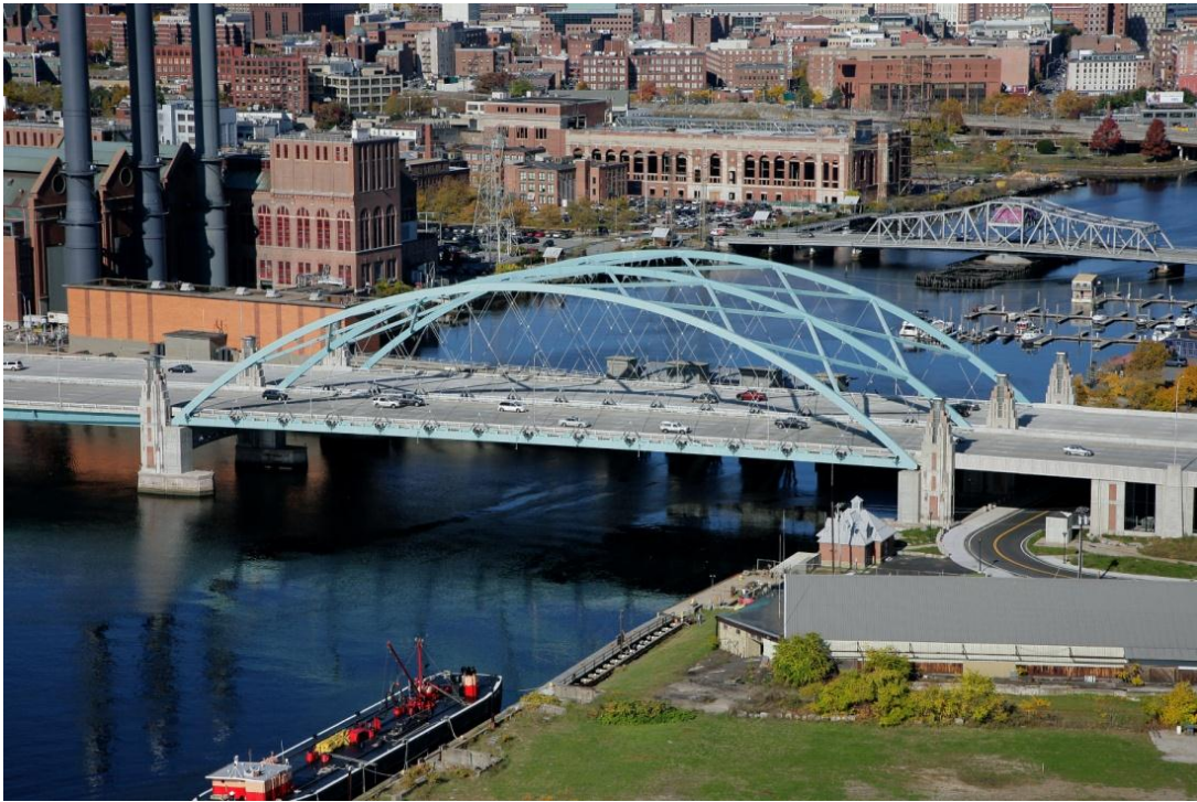
Fig. 29. The network arch in Providence, Rhode Island, USA. Opened 2007. Span of 122 m.
