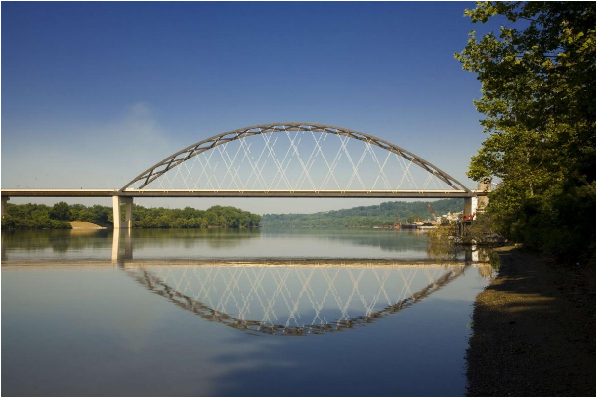
Fig. 32 Blennerhassett Bridge over the Ohio River was opened in 2008. Span 267.8 m.
