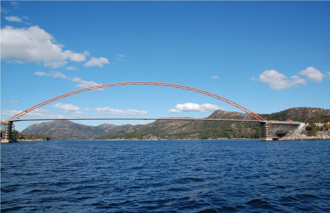
Fig. 23 shows the Brandanger Bridge before the railings were erected
