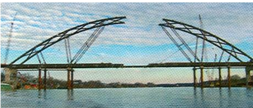
Fig. 34. Erection of the Blennerhassett Bridge
