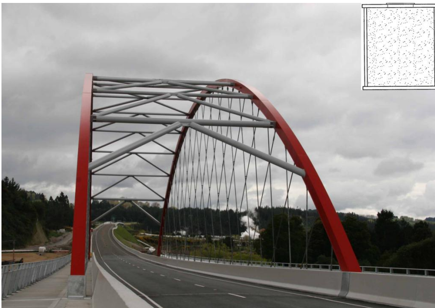
Fig. 28. Waikato River Bridge was opened in New Zealand in 2011. Span 100 m.
