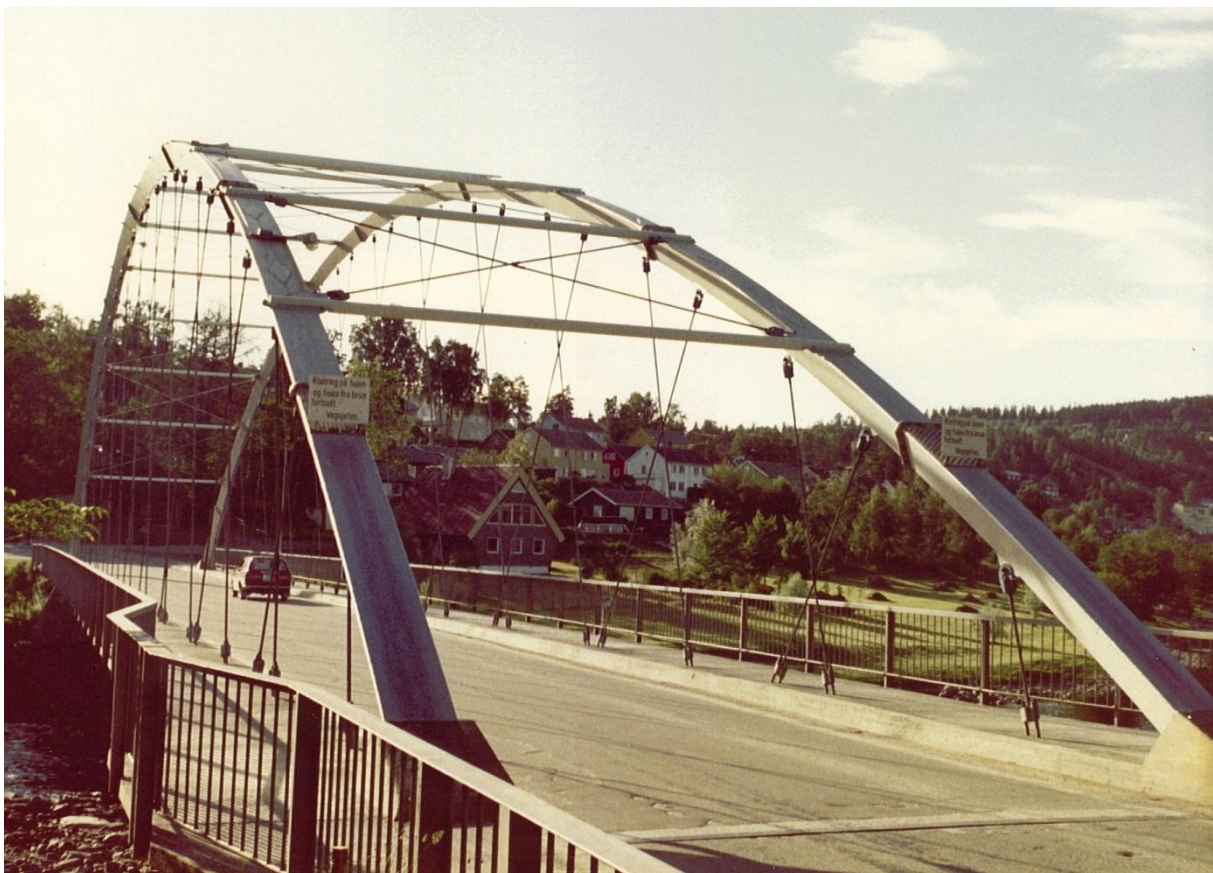
Fig 1. The first Network Arch opened at Steinkjer in 1963. Span 80m (Tveit 1964)
