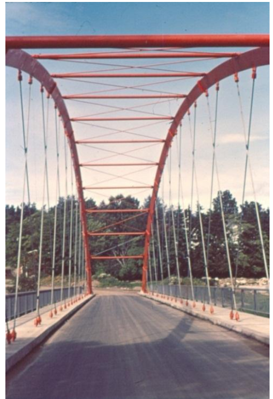
Fig. 4 The network arch looked like this before it got its final coat of paint.
