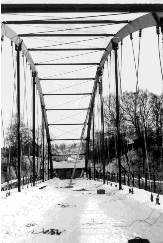
Fig. 12 shows the erection in the winter of 1963
