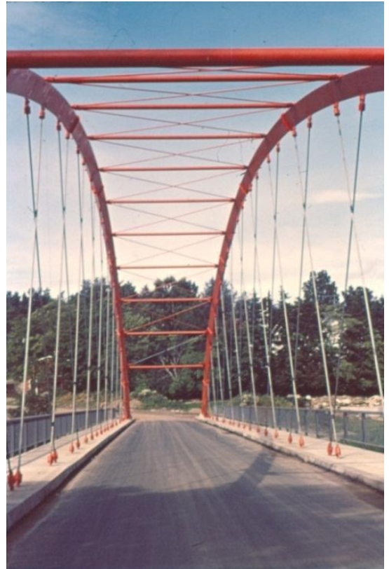
Fig. 4 The network arch looked like this before it got its final coat of paint.
