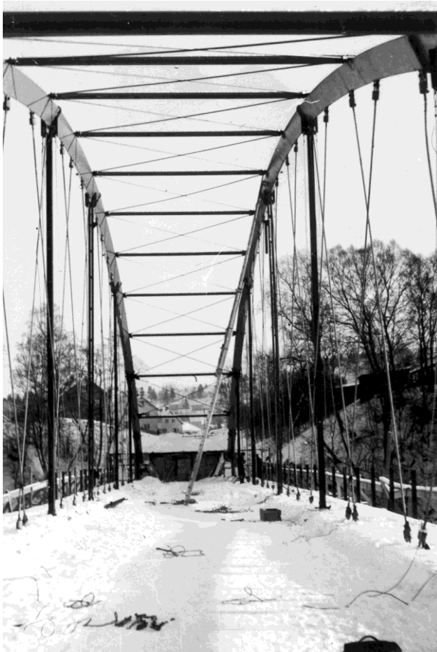
Fig. 12 shows the erection in the winter of 1963
