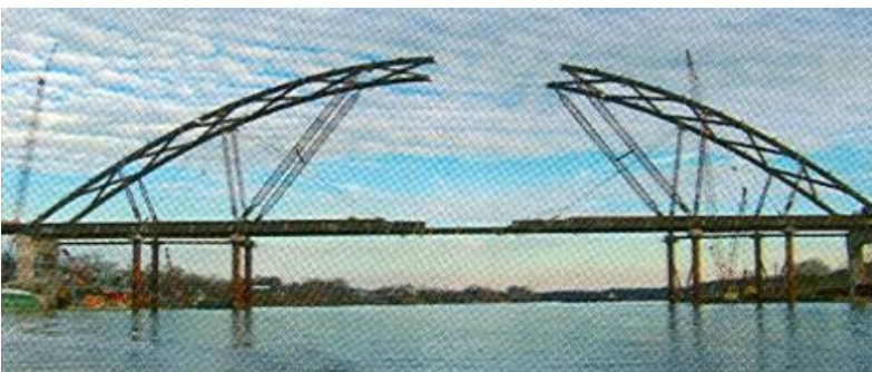
Fig. 34. Erection of the Blennerhassett Bridge
