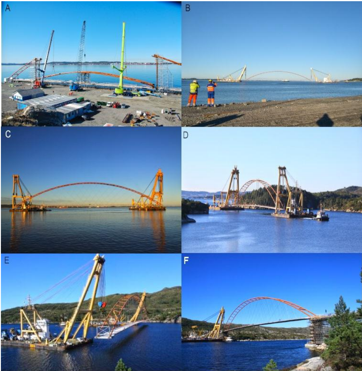
Fig. 25 A: Building of the main span 5 km from the site
