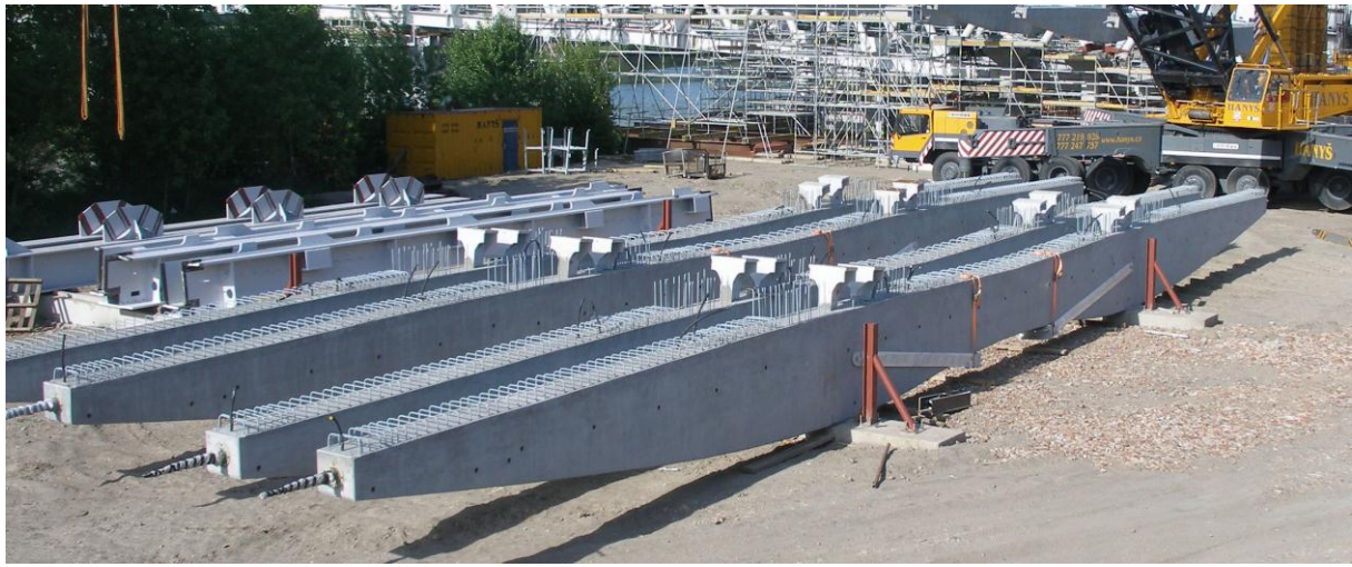
Fig. 4 Precast transversal beams stored on the site prior to assembly
