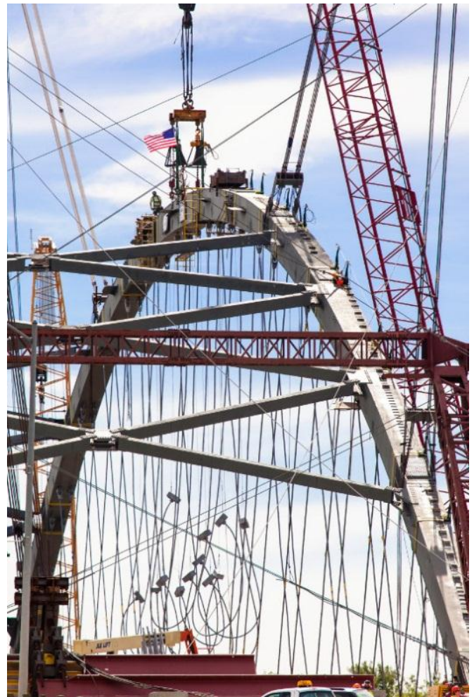
Figure 5 – Erection of the Arch Keystone Piece
