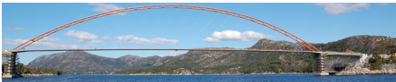
Fig. J13. The Brandanger network arch in western Norway. Span 220 m. Opened 2010
