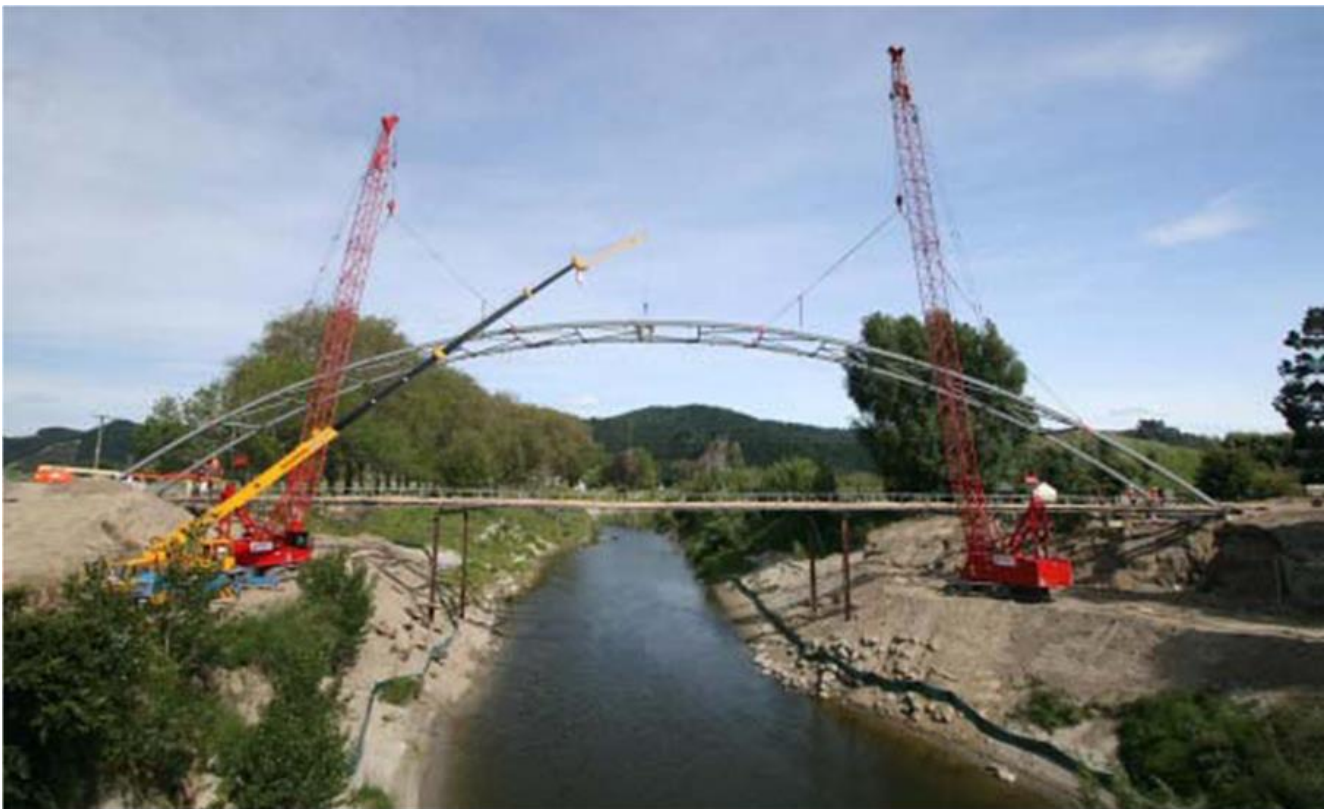
Fig. E8. Method for lifting the steel skeleton of the Mangamahu Bridge in place. Span 86 m. Built 2008.
