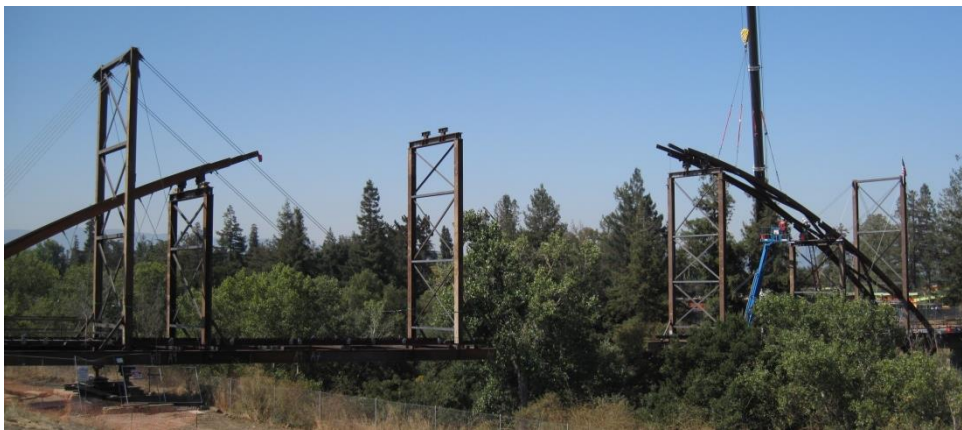
Figure 8 - East Arch Erection
