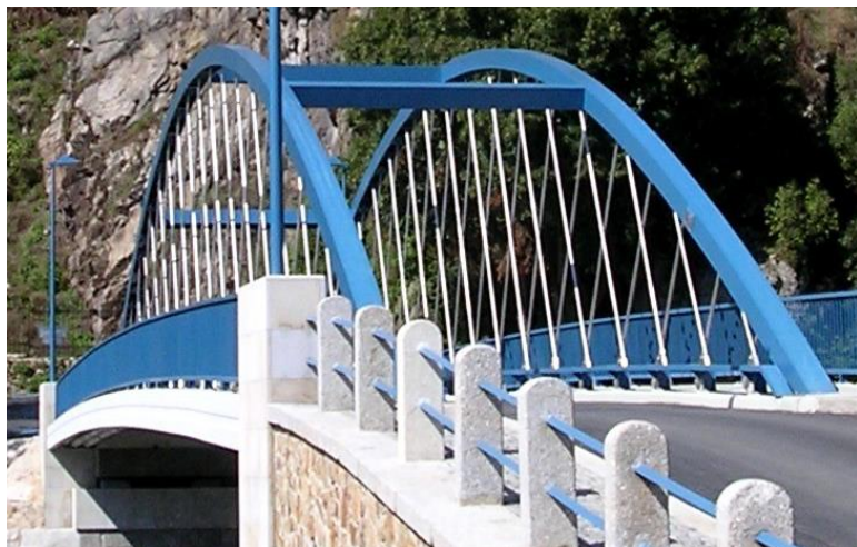
Fig. 1. Approach to the Bechyň Bridge
