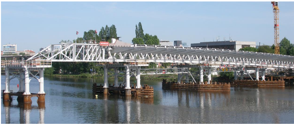
Incremental launching of the steel truss and precast transversal beams
