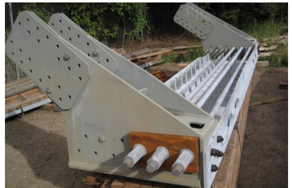
Figure 5 - Knuckle Joint
