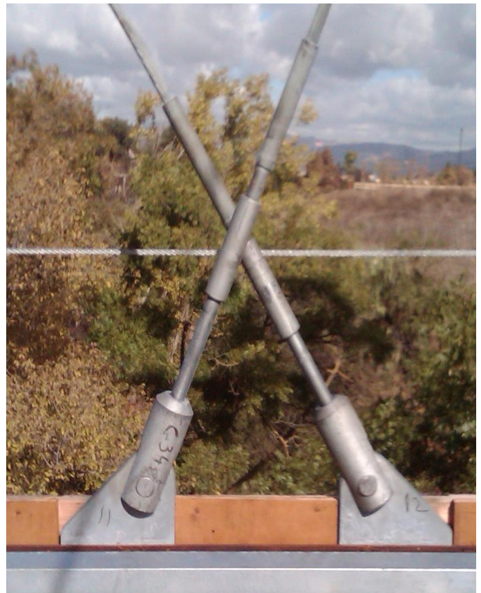
Figure 6 - Lower Hanger Connections
