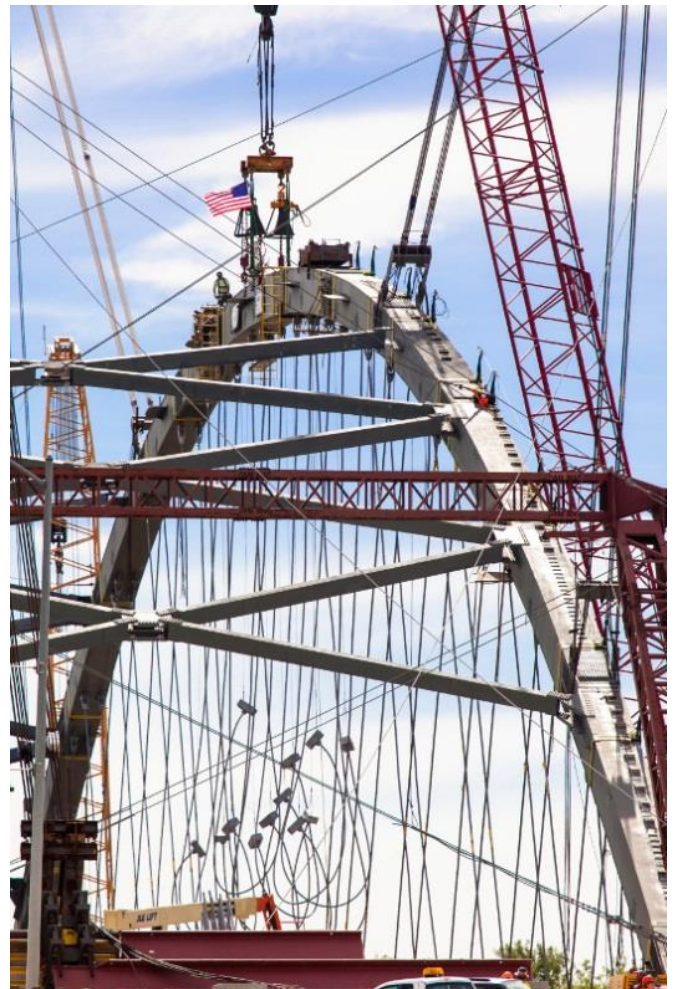
Figure 5 – Erection of the Arch Keystone Piece
