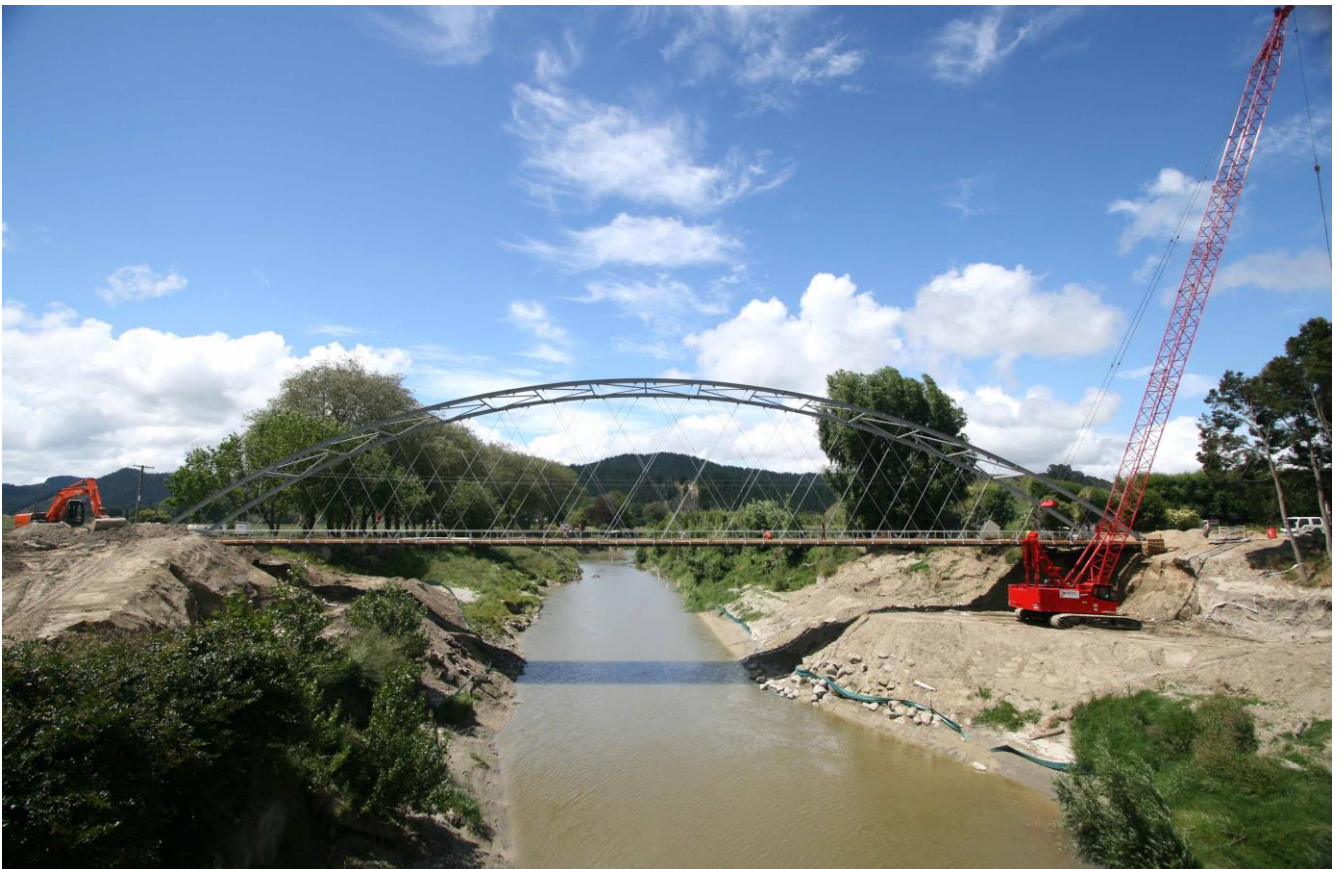
Fig. J20. Steel skeleton of the Mangamahu network arch that was lifted in place by mobile cranes
