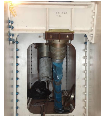
Fig. 6 – Cable Anchorage in Tie Girder
