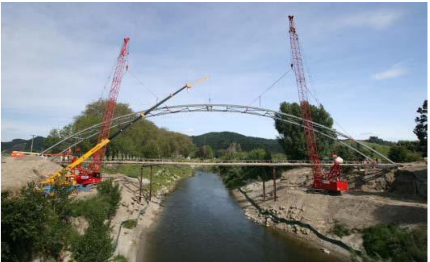
Figure 4 - Erection of the arches with mobile cranes
