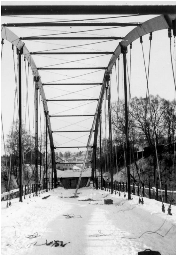
Fig. J9. Erection of arch and hangers at Steinkjer in the winter of 1962-1963
