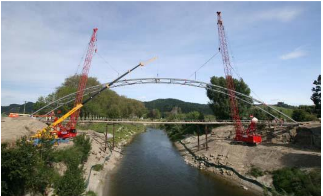
Figure 4 - Erection of the arches with mobile cranes
