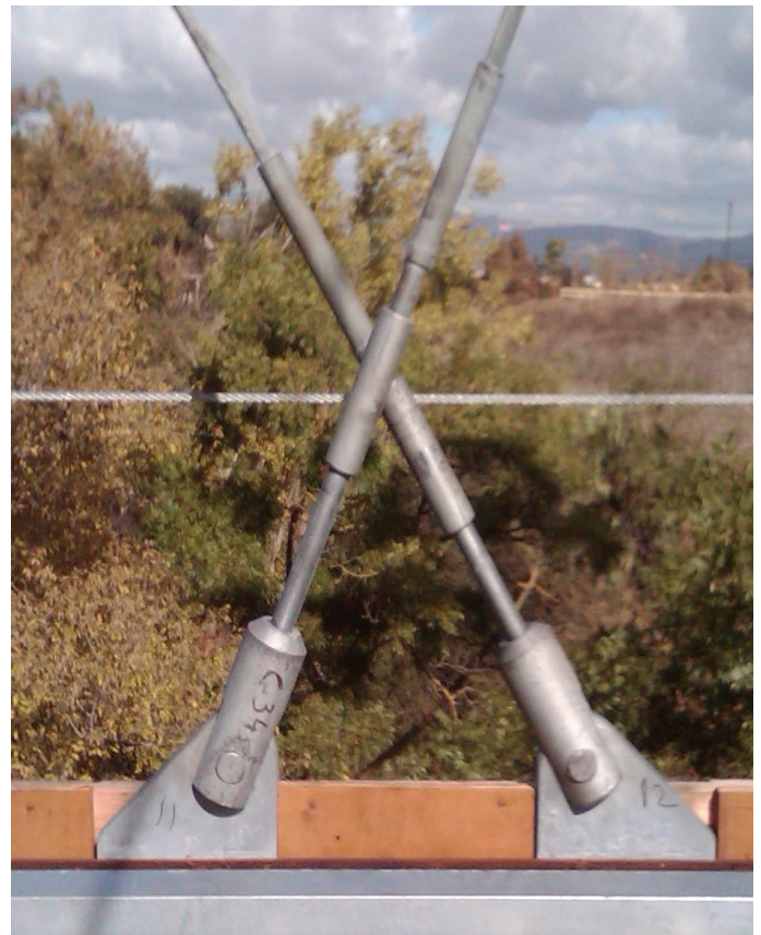
Figure 6 - Lower Hanger Connections
