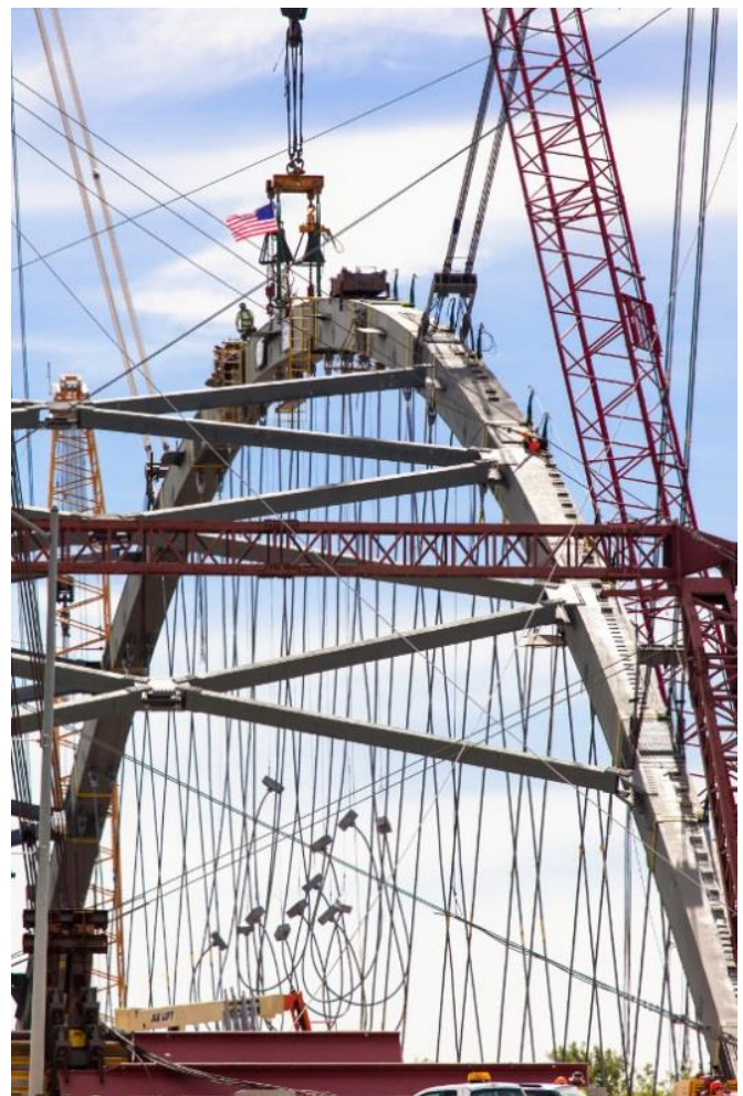
Figure 5 – Erection of the Arch Keystone Piece
