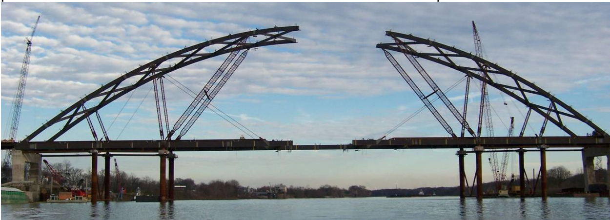
Fig. 8 – Arch Erection
