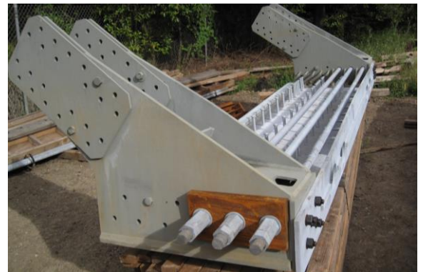
Figure 5 - Knuckle Joint
