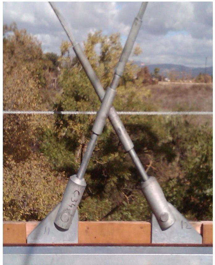
Figure 6 - Lower Hanger Connections
