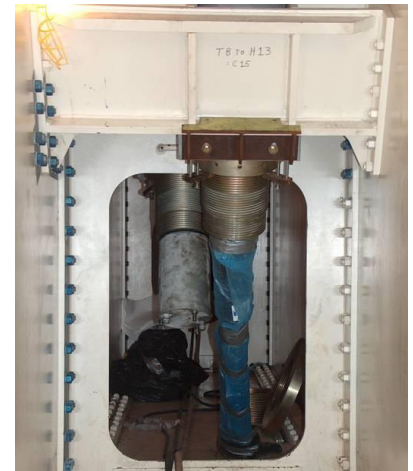
Fig. 6 – Cable Anchorage in Tie Girder
