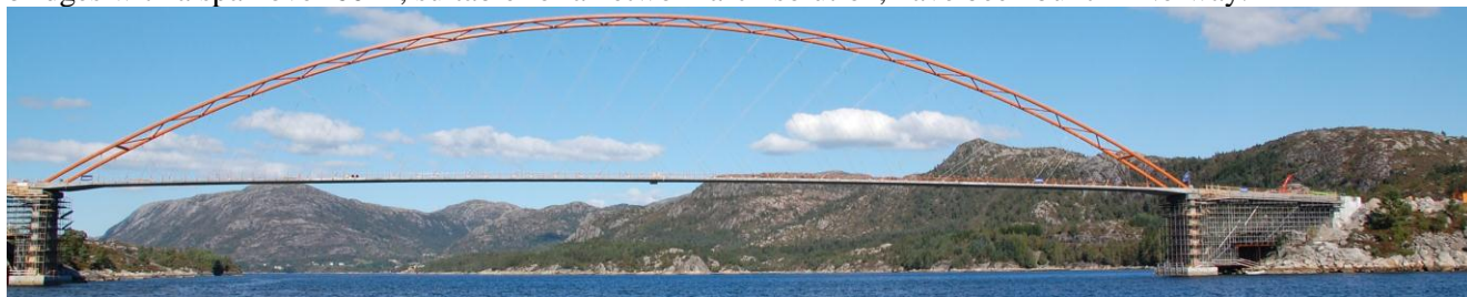
Fig. J12a. The Brandanger network arch in western Norway. Span 220 m. Opened 2010
