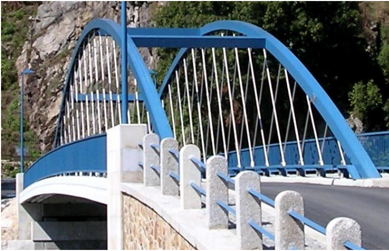
Fig. 1. Approach to the Bechyne Bridge
