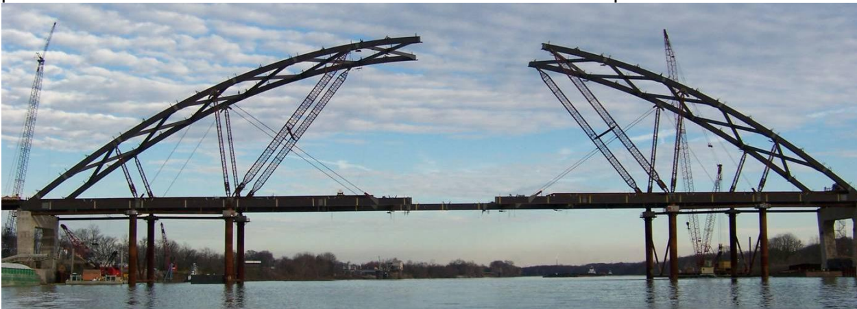
Fig. 8 – Arch Erection
