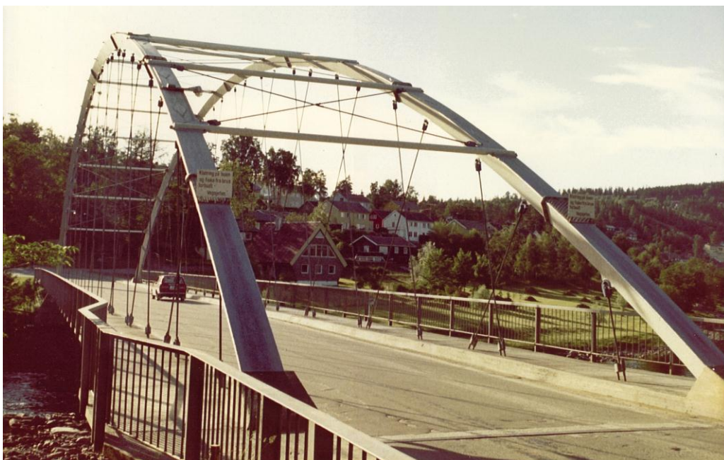
Fig. J10. The finished network arch at Steinkjer, Norway. (Photo Alvestrand)
