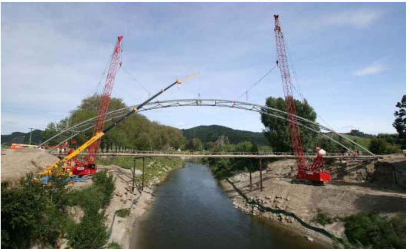
Figure 4 - Erection of the arches with mobile cranes
