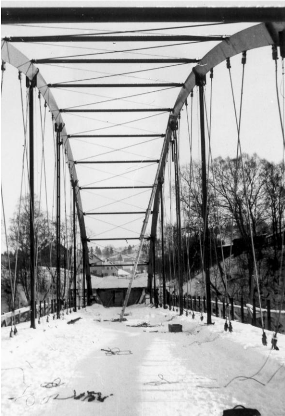
Fig. J9. Erection of arch and hangers at Steinkjer in the winter of 1962-1963
