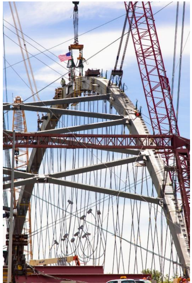
Figure 5 – Erection of the Arch Keystone Piece
