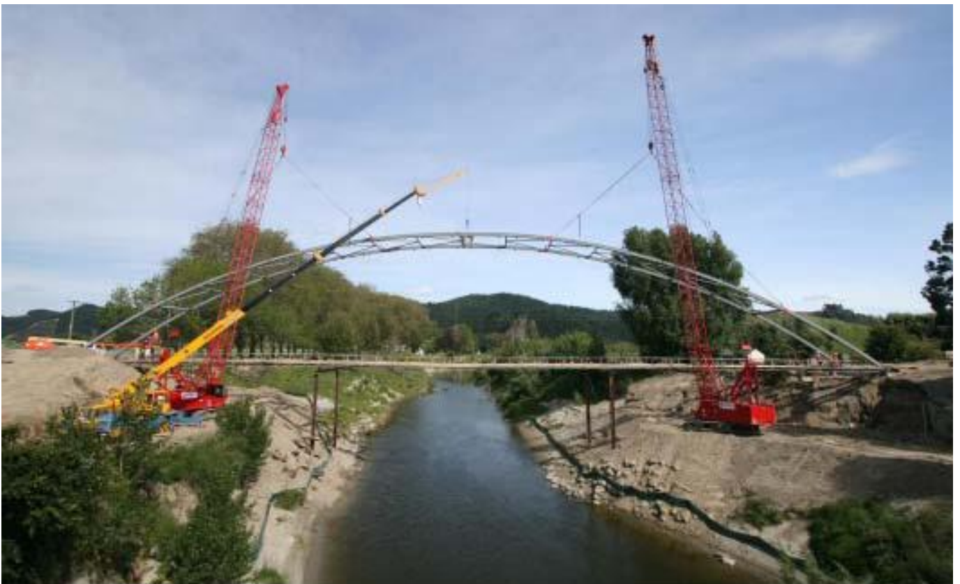
Figure 4 - Erection of the arches with mobile cranes
