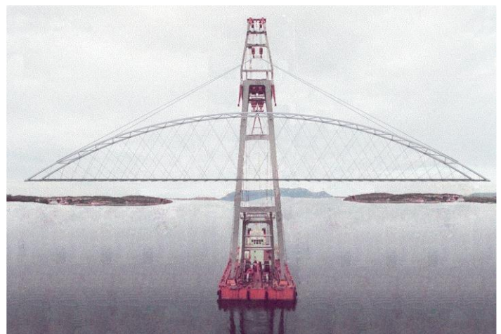
Fig. E10. Lifting the temporary steel skeleton of the bridge in Fig. C1
