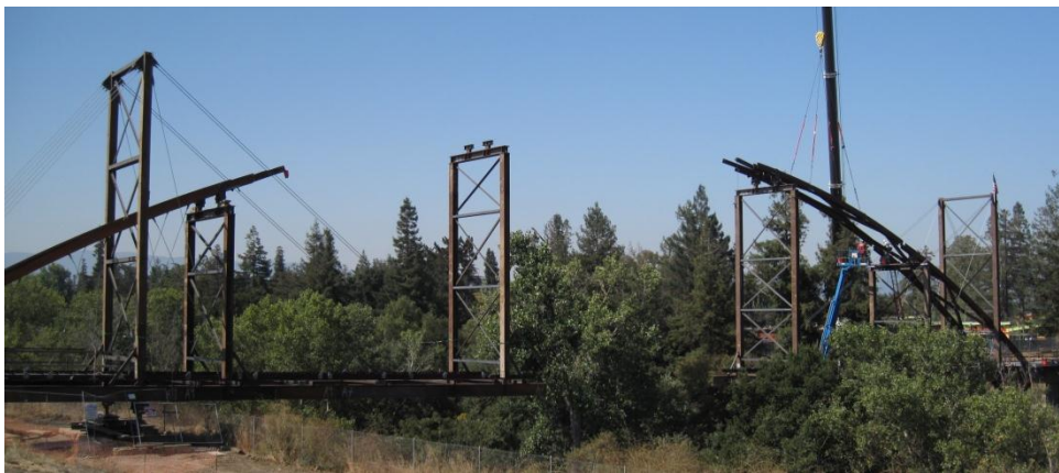
Figure 8 - East Arch Erection
