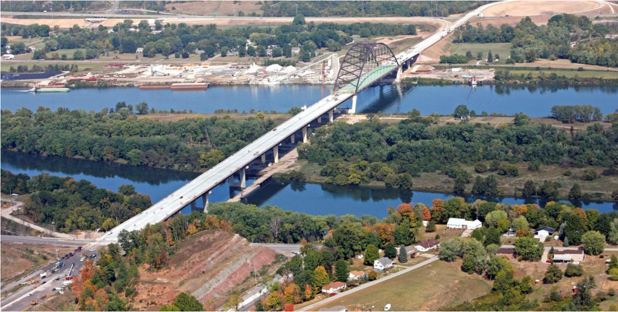
Fig. 1 – Blennerhassett Island Bridge
