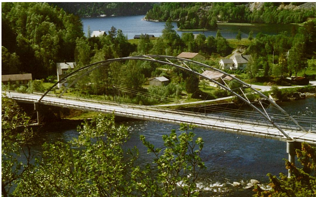
Fig. 7. Bolstadstraumen Bridge. The main span is 84 metres.
