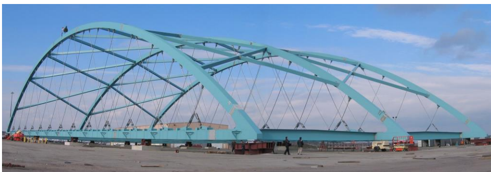
Fig. 31a shows the steel skeleton of the network arch at Providence before it is floated to the site
