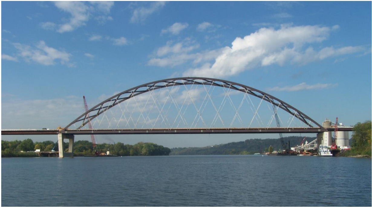
Fig. 31b. Bridge over the Ohio River in the USA. Opened 2007. Span 268 m.
