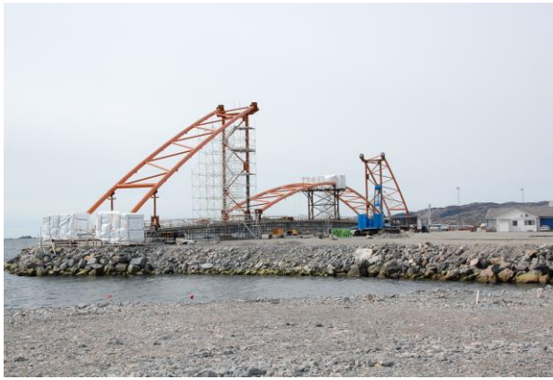
Fig. 102. Stage in the building of the main span.
