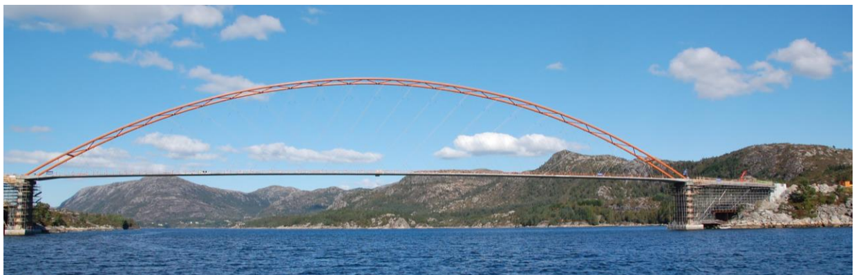
Fig. 101. The Brandanger Sound Bridge was lifted onto the pillars on the 7th of September 2010
