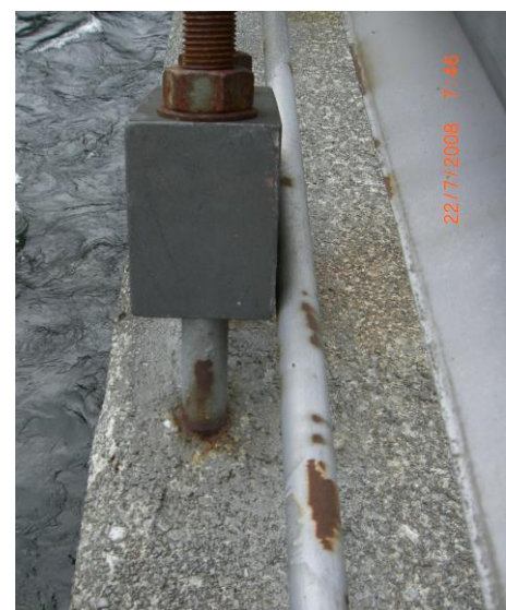
Fig. 61g and fig. 61h. Lower ends of hangers coming out of concrete in the Bolstadstraumen Bridge
