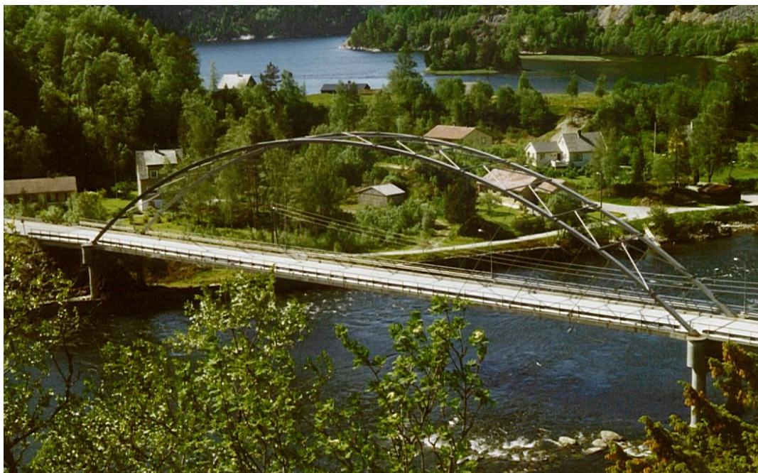
Fig. 7. Bolstadstraumen Bridge. The main span is 84 metres.
