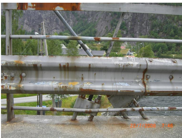
Fig. 61g and fig. 61h. Lower ends of hangers coming out of concrete in the Bolstadstraumen Bridge
