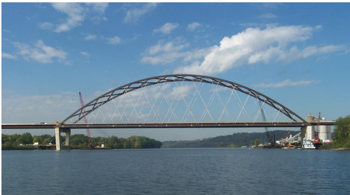
Fig. 31b. Bridge over the Ohio River in the USA. Opened 2007. Span 268 m.
