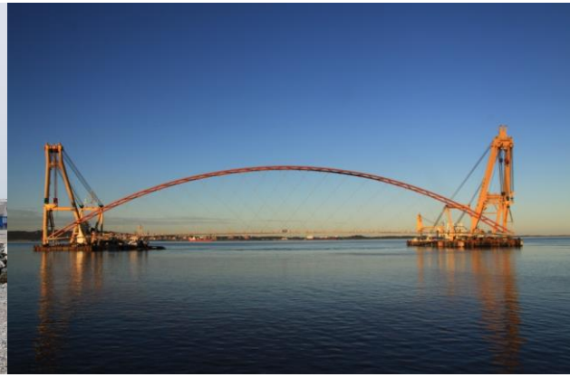
Fig. 103. Brandanger Bridge. Transport of the main span.
