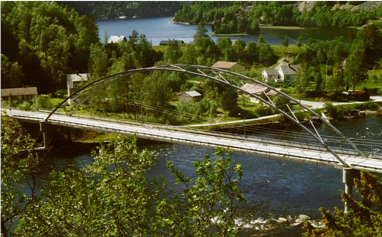
Fig. 6. The Bolstadstraumen network arch in western Norway was opened at the end of 1963. Span 84 m.
