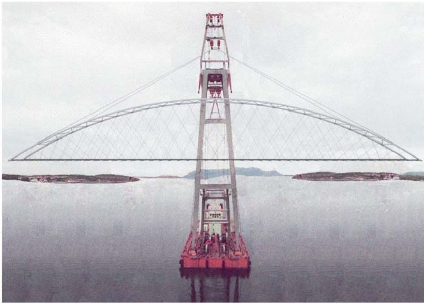
Fig. 18. Lifting of the steel skeleton of the Åkvik Sound Bridge
